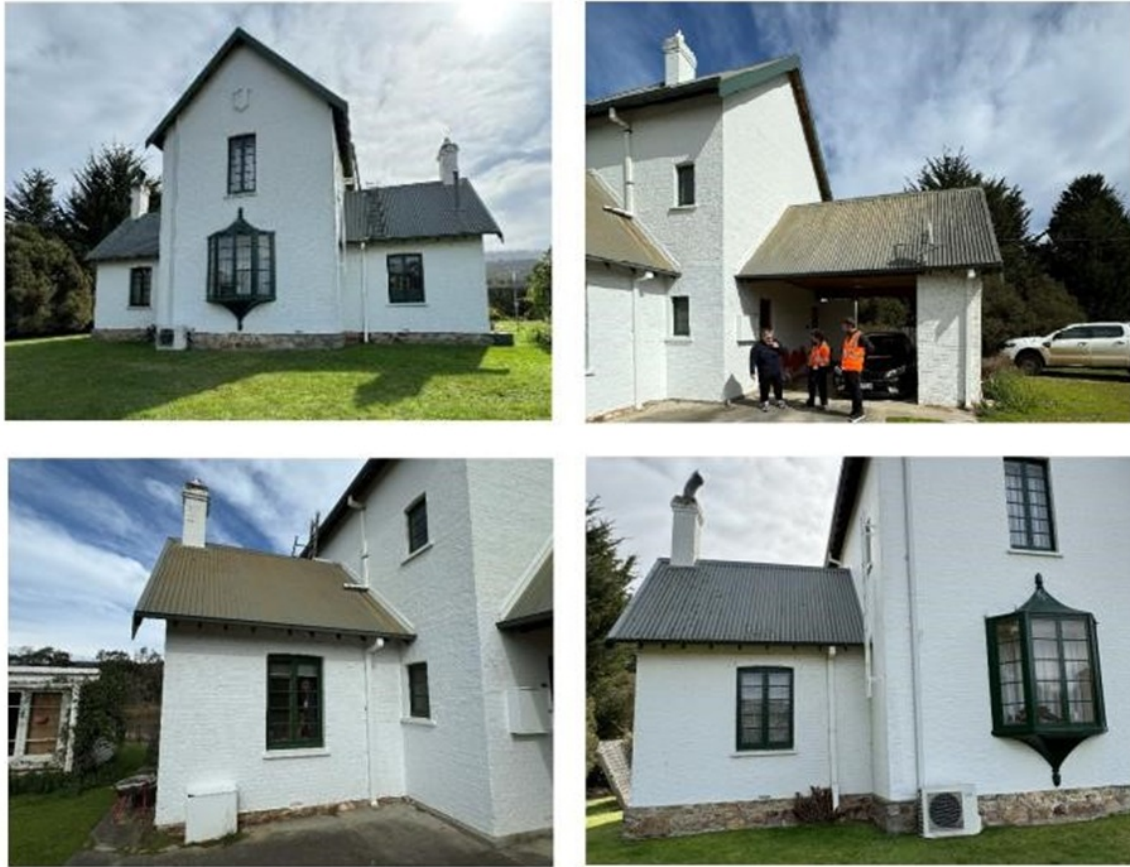
Figure 7, Figure 8, Figure 9 and Figure 10 - External views of The Grange (September 2024) - source: John Wadsley. Top left: Southern side with oriel window; note the original shield above the first-floor window, Top right: Northern side with carport added in 1969, Bottom left: Eastern wing from northern side, Bottom right: Western wing from southern side.
