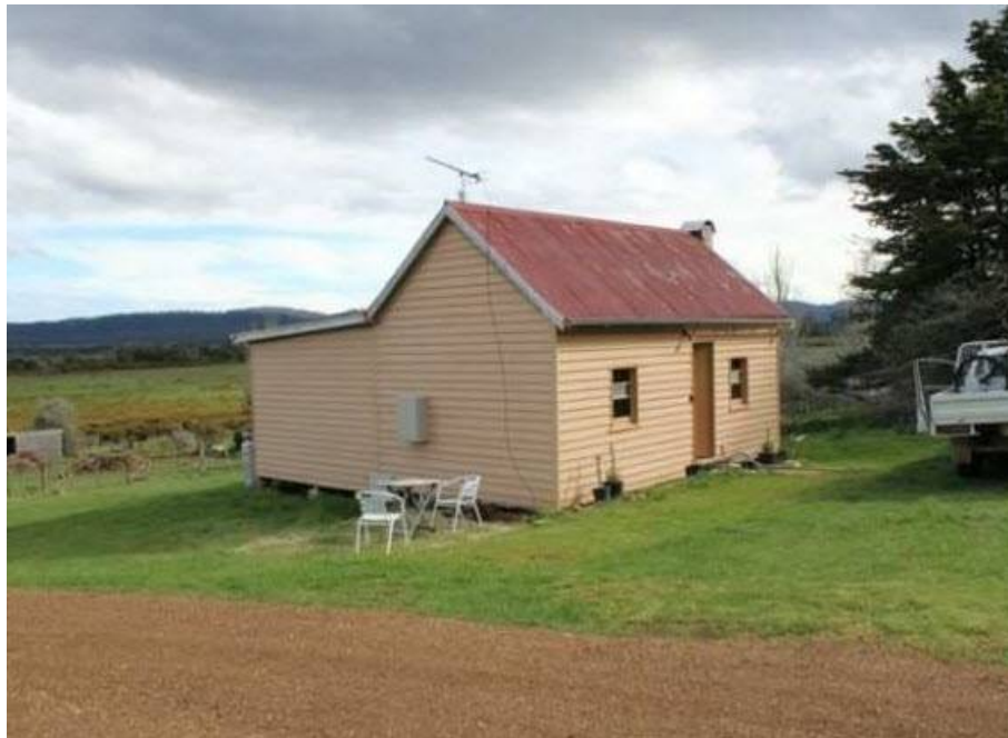
Figure 7: View of ancillary dwelling
