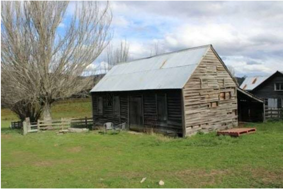
Figure 6: View of Barn from the North
