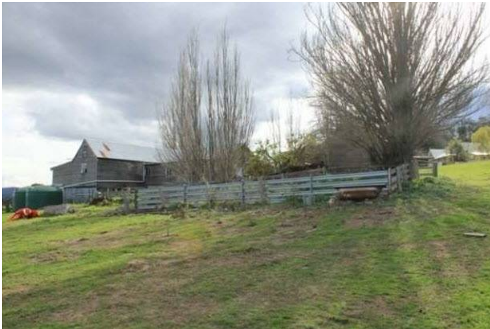
Figure 5: View of Shearing Shed from the East
