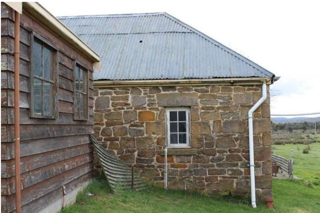
Figure 4: Rear outbuilding of stone construction with hip roof
