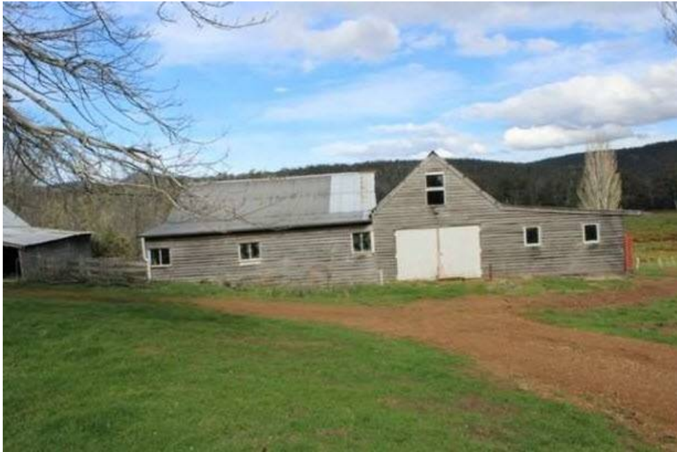
Figure 4: View of Shearing Shed from the West
