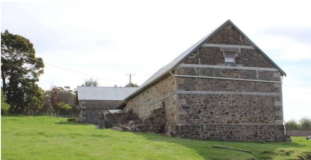
Figure 3: View of rear West façade of Stables building and annex
