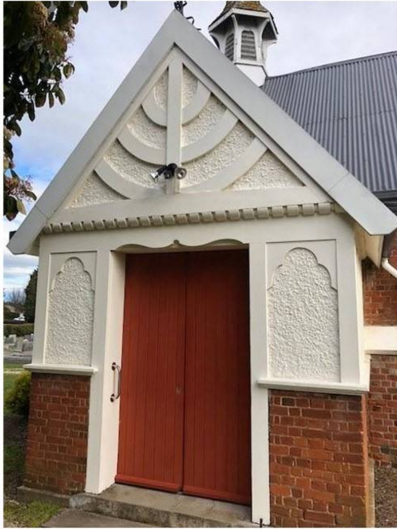
Entrance with decorative timber detailing to gable end and upper section of walls
