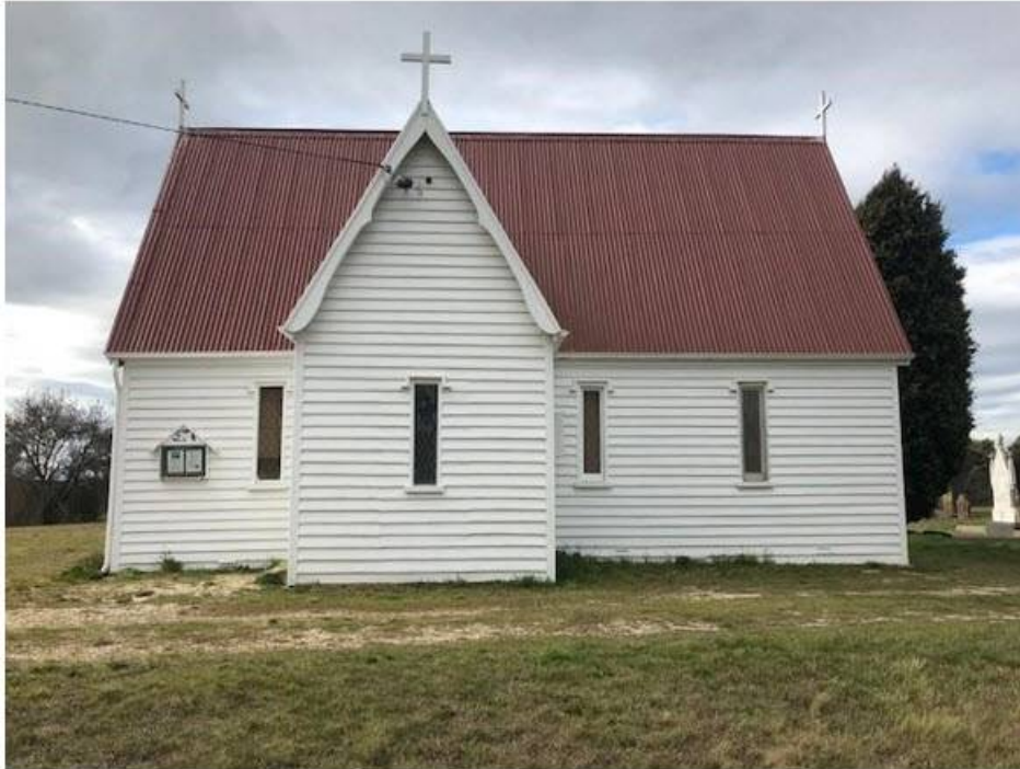
Figure: South side of the building showing the small gable roof wing and narrow window
