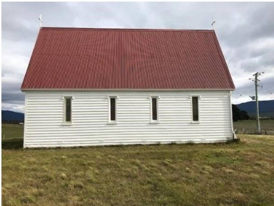
Figure: North side of the building with 4 equally spaced narrow windows. The weatherboards extend to the ground with no visible foundation wall
