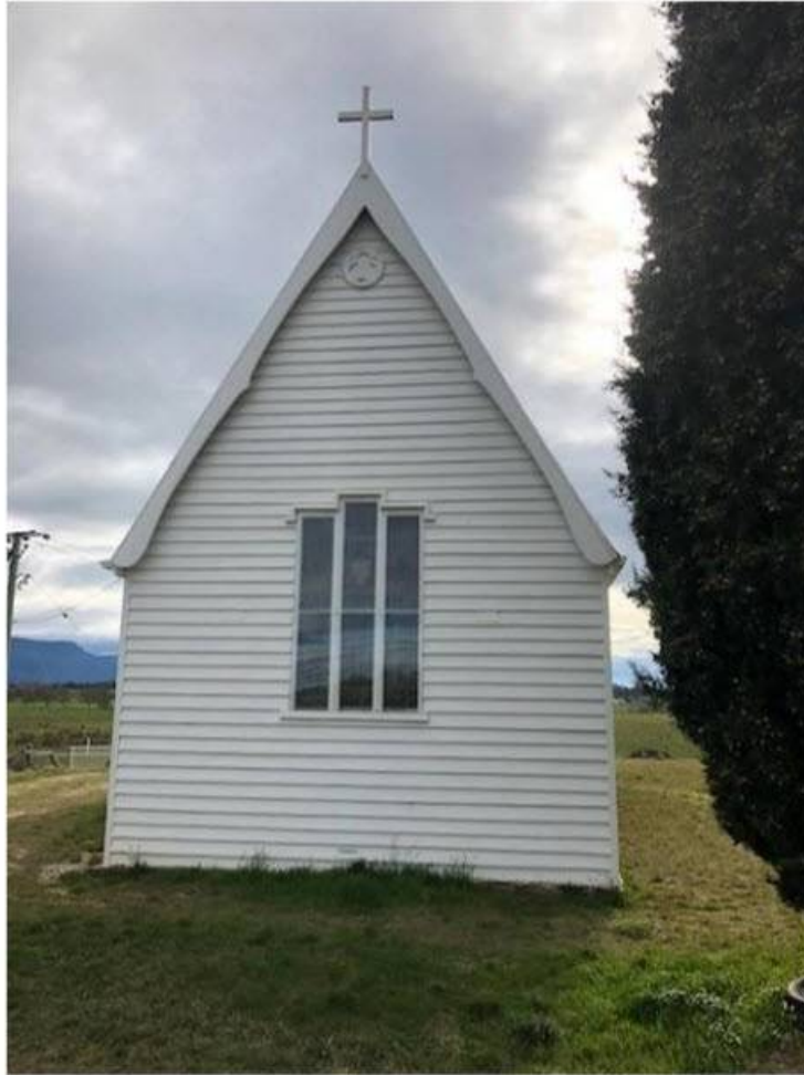
Figure: East side of the building showing the steep gable roof with modestly shaped barge boards and narrow window frames. The narrow windows forms have been coupled together to form a wider window.
