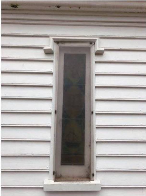
Figure: View of narrow side window with bottom beaded timber weatherboards
