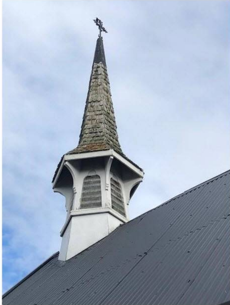
Hexangular Belfry with timber louvre bell screen, huon pine shingle roof and decorative iron finial
